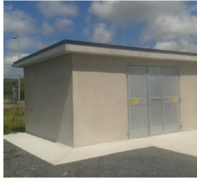
Fig. 1: Freestanding MV substation.
