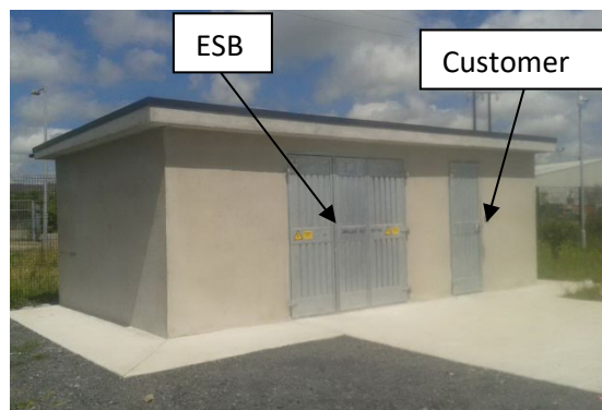
Fig. 2: Freestanding MV substation adjoining a customer's switchroom.
